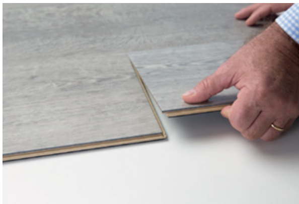
05: Continue pressing until you hear the "Click" sound of the drop-click lock system
